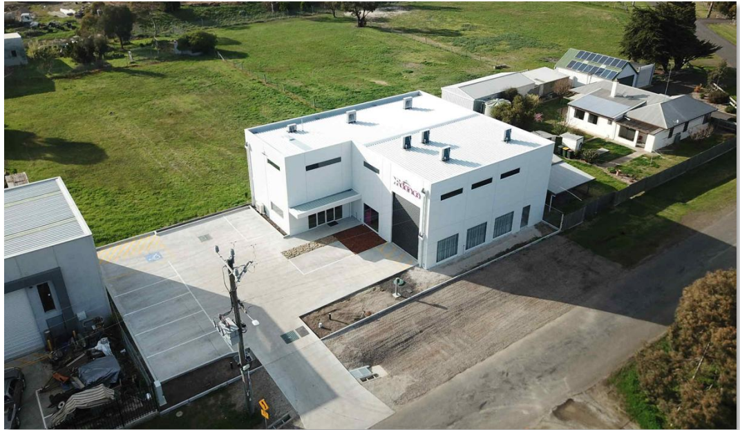
Subject site | Aerial view
